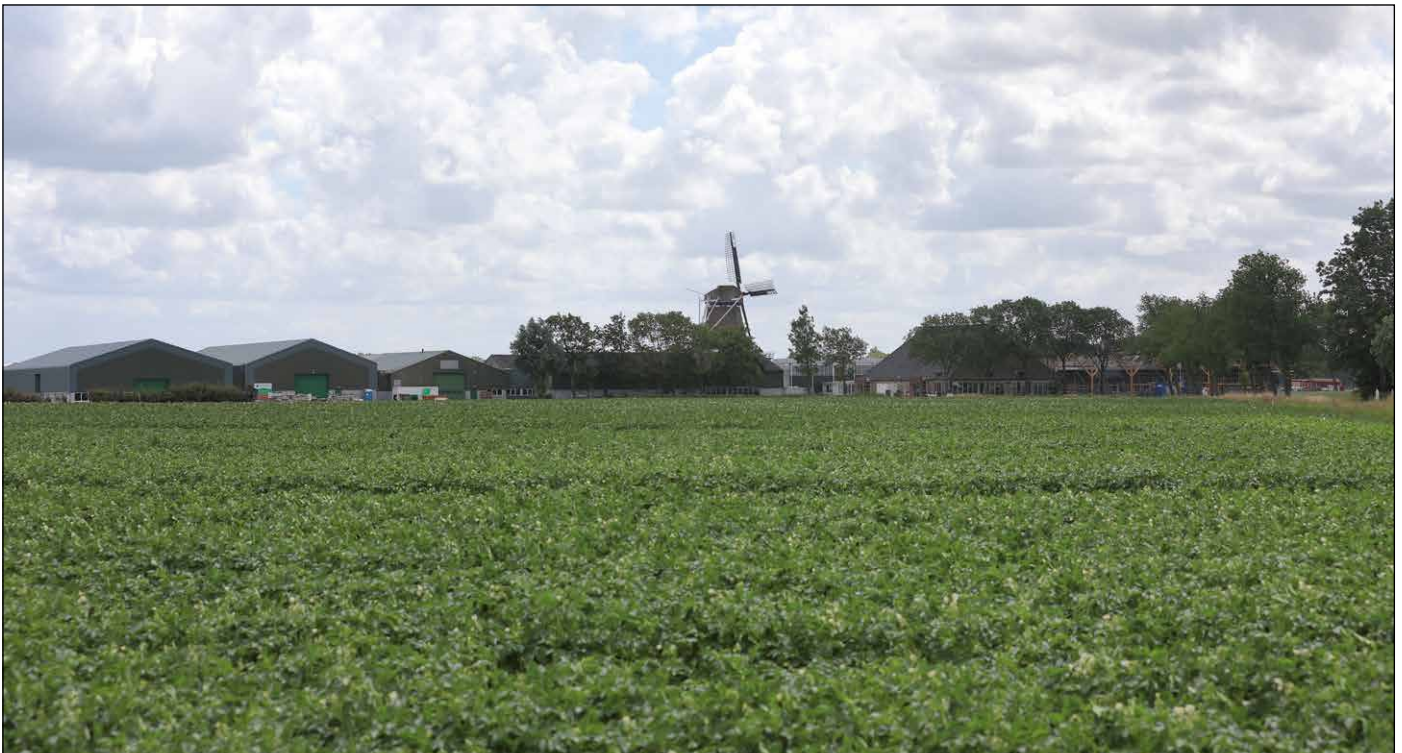
Contractors are busy expanding and modernising the buildings of HZPC Research.
